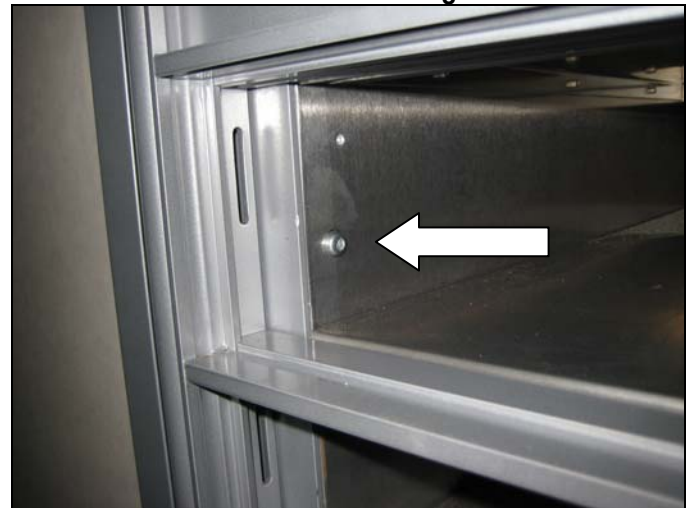
Illustration 3 - Location of Mounting Hardware Hole
